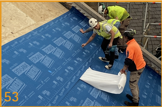
Place and Adhere Course by Course SOLITEX EXTASANA ADHERO may be rolled out course by course on roofs above 5° pitch.
