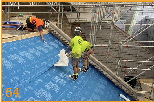
Overlap, Remove Backing and Adhere Overlapping joints by 150mm, remove backing and adhering in same method as for low pitch roofs. No primer in joints is necessary for roof >5° pitch.
