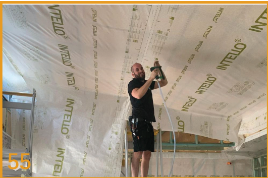
Apply INTELLO® PLUS INTELLO® PLUS Intelligent Air Barrier should be installed to the underside of the fibrous insulated roof structure in accordance with pro clima's instructions.
