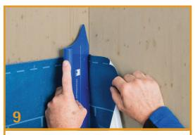
**Apply Membrane Without Internal Corner** To form the corner, guide at least 150 mm of the membrane around the corner. Apply pressure and smooth ADHERO® using PRESSFIX XL.
