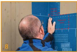
Adhere only the 200 - 300 mm released part of the application zone. Ensure that the membrane covers at least 150 mm of the corner strip.
