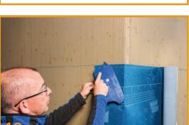
**Apply Membrane Without External Corner** Wrap SOLITEX EXTASANA ADHERO® at least 150 mm around external corners. Apply pressure and smooth ADHERO® using PRESSFIX XL.
