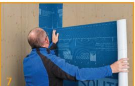
Apply Membrane to Align with Internal Corner Remove approx. 200 - 300 mm of the release film of the upper application zone. Position the membrane at the marking (on the wall) and attach to the wall.
