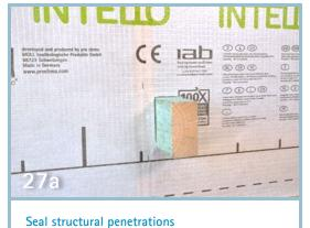
Cut INTELLO® flush with the sides. Seal the bottom side first. Cut a length of TESCON® PROFIL 60 mm longer than the narrow side.
