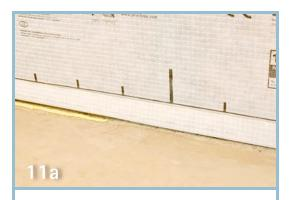
Apply ORCON® CLASSIC bead along floor Hold the INTELLO® overlap up & apply a bead of ORCON® CLASSIC adhesive that is at least 5 mm thick along the floor (concrete, fc sheet or timber).
