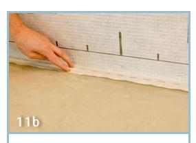
Attach INTELLO® to ORCON® CLASSIC bead Lay the INTELLO® overlap onto the ORCON® CLASSIC bead in full contact. Do not press the bead completely flat, allowing a lasting, flexible connection.
