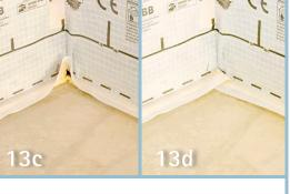
Pinch any extra INTELLO® material and lift it up. continuous seal.
