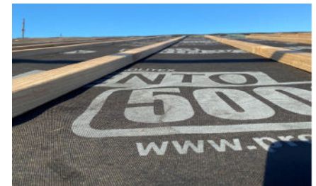
Figure 13: With purpose-built cavity the counter battens define the ventilation cross-sectional area. The type of cladding, metal or tiles is therefore irrelevant and only changes the batten spacing. (Image: Pro Clima Australia)
