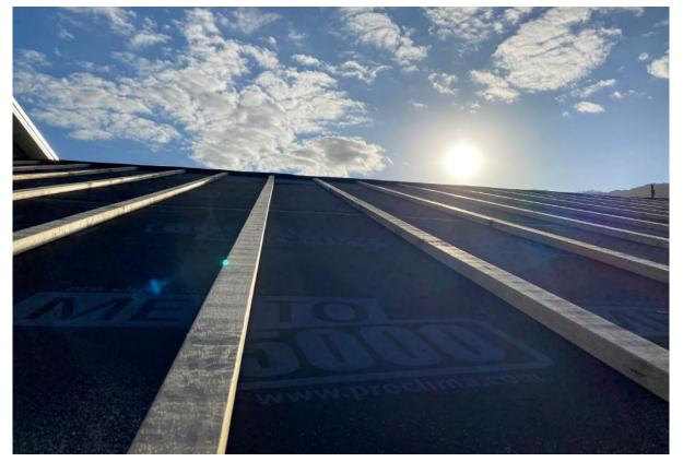
With up to 180 days UV exposure prior to cladding and more than 100°C continuous operating temperature SOLITEX® products are built to last in the harshest summer conditions.
