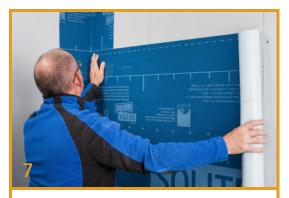
Apply Membrane to Align with Internal Corner Remove approx. 200 – 300 mm of the release film of the upper application zone. Position the membrane at the marking (on the wall) and attach to the wall.
