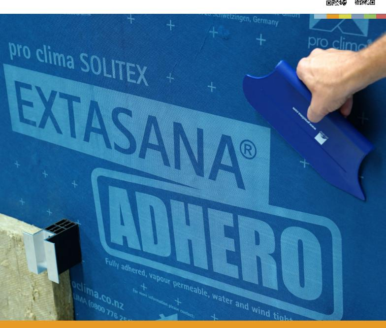
Self-Adhesive Weather Resistive Barrier for Walls and Roofs
