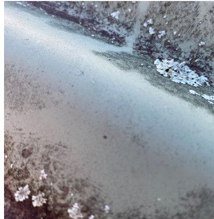
Figure 6: Over time the absorptivity of the roof will increase as the roof ages, surfaces dull and dirt, grime and lichens accumulate. (Image: Jesse Clarke, Pro Clima Australia)
