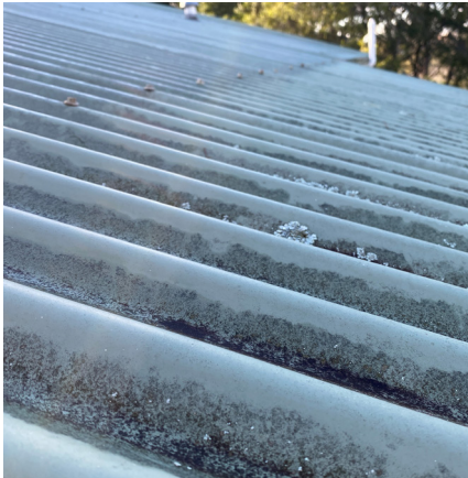
Figure 6: Over time the absorptivity of the roof will increase as the roof ages, surfaces dull and dirt, grime and lichens accumulate. (Image: Jesse Clarke, Pro Clima Australia)
