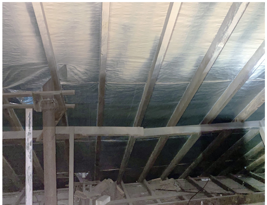
Figure 4: Foil has become engrained in the psyche of the Australian building industry as a one-sided solution to improve summer performance of buildings. But installing a vapour barrier, such as foil, can lead to perverse outcomes during winter. (Image: Sean Maxwell)
