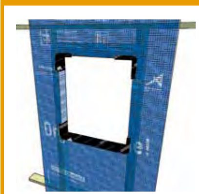
Apply TESCON EXTORSEAL sill tape to wall openings as per NZBC Acceptable Solution E2/AS1 paragraph 9.1.5.
