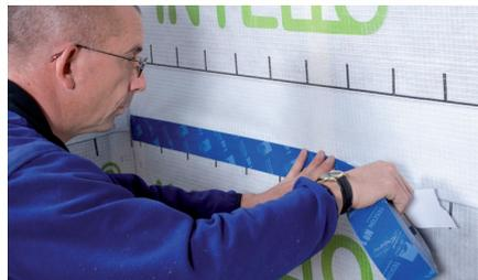
Seal the membranes at overlaps without strain or loading, using TESCON® VANA adhesive tape. The tape should be applied centrally and pressed down firmly using, for example, pro clima PRESSFIX.
