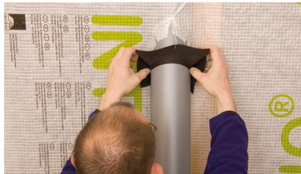
ROFLEX pipe grommets are affixed using TESCON® EXTORA. Press firmly to secure the adhesive tape.
