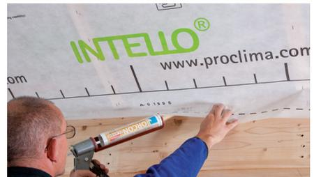
The liquid adhesive ORCON is applied to join the INTELLO® membrane to concrete or wooden frames. Do not press the adhesive completely flat.
