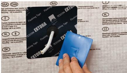
If pipes or cables penetrate the airtightness layer, they too must be securely sealed. KAFLEX cable grommets are self-adhesive. Remove the release paper, push over the cable and stick on.
