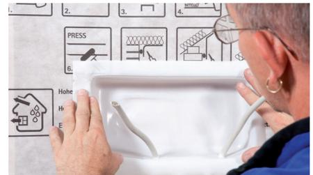
The airtightness box for power points and light switches is cut and fitted into the INTELLO® layer and then sealed by using TESCON® VANA to create a seamless airtightness system.
