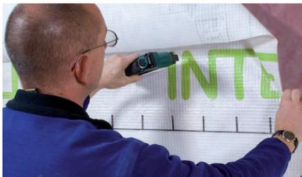
The INTELLO® airtightness membrane is laid on the interior, over the insulation. Bonding with adhesive tapes should be on the smooth printed side. Staples should be 10 mm wide and 8 mm long and set at a max distance of 100 mm - 150 mm.
