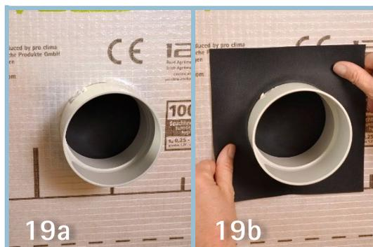
**Sealing large pipes using ROFLEX**
