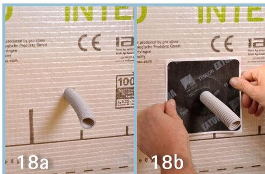
**For small pipes use ROFLEX 20 grommet**
