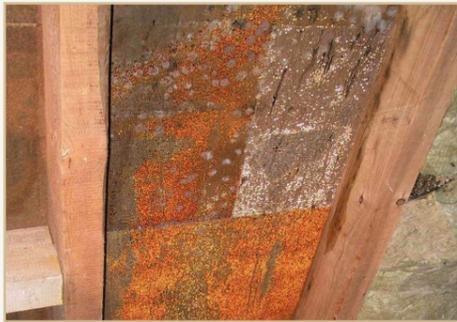
Without moisture management there is a risk of water condensing in the building envelope, and thus a risk of structural damage and mould.
