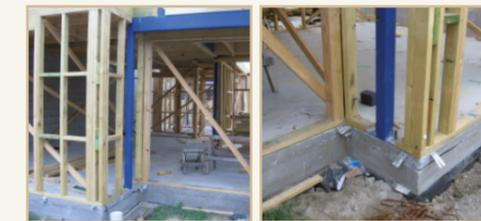
Insulate steel beams on at least one side, preferably on the outside
