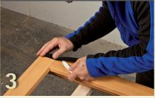
Remove the backing paper, align the tape straight on the frame and gradually stick in place. The tape must not be visible after installation (recess approx. 1 - 2 mm).
