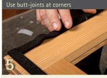
Stick the tape around the circumference of the frame. Use one length of CONTEGA FIDEN EXO per side here and use butt-joints at the corners. Allow for a small amount of slack near the corners.
