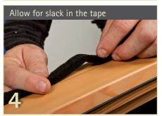
Allow for a small amount of slack in the tape when sticking it in place, particularly near joints – **do not stretch the tape!**
