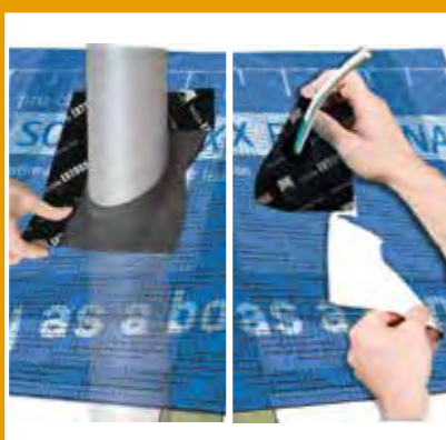
Use pro clima ROFLEX to seal pipe penetrations as per Acceptable Solution E2/AS1 paragraph 9.1.9.3. and pro clima KAFLEX for cable penetrations.
