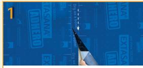
Remove both release papers and adhere from top down following a pre-marked vertical line.
