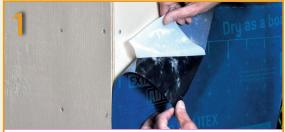
Remove 150mm release paper and adhere to substrate on a pre-marked height.
