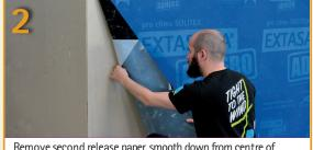
Remove second release paper, smooth down from centre of sheet working outward. Use PRESSFIX-XL Overlap minimum 150mm as per markings. Must extend over the bottom plate by minimum 35mm.
