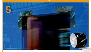
Apply TESCON EXTOSEAL sill tape to wall openings as per NZBC Acceptable Solution E2/AS1 paragraph 9.1.5.b.
