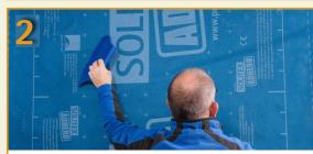
Overlap by min 150mm at vertical joins, smoothing down underlay evenly across the sheet width using PRESSFIX-XL. Must extend over the bottom plate by minimum 35 mm.
