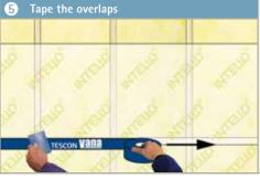
Tape the INTELLO® PLUS with TESCON VANA adhesive tape so that it is free of any tension or stress. Position the tape centrally and press firmly to secure using the PRESSFIX. Cut a slit in any folds in the overlapping part of the membrane and re-tape.
