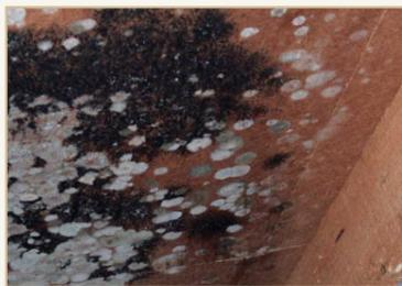
Constructions that are not airtight do not only result in mould on the inner surfaces of structural components, but also in mould within the construction.
