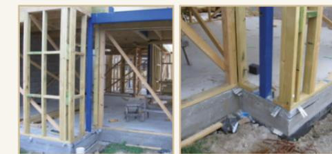
Insulate steel beams on at least one side, preferably on the outside
