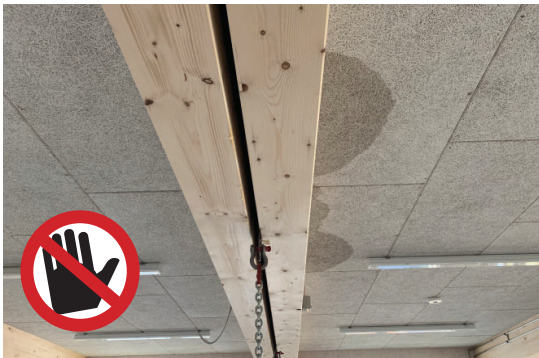
Leaky module joint
