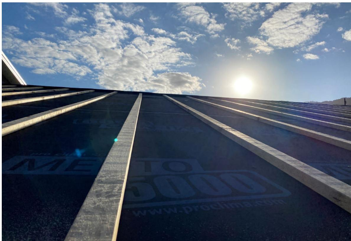
With up to 180 days UV exposure prior to cladding and more than 100°C continuous operating temperature SOLITEX® products are built to last in the harshest summer conditions.
