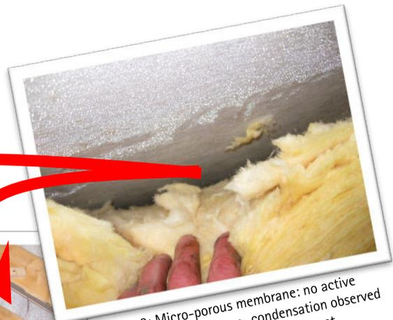
Figure 2: Micro-porous membrane: no active vapour transportation -> condensation observed and creates a vapour closed film -> wet construction
